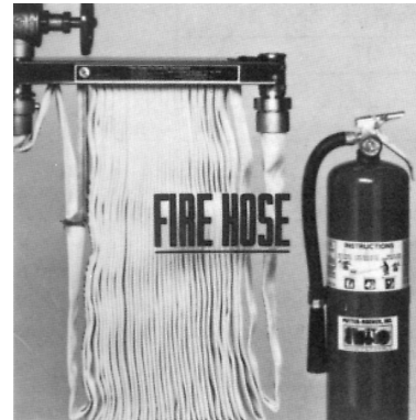
FIGURE A.3.3.16.4 Semiautomatic Hose Rack Assembly.
